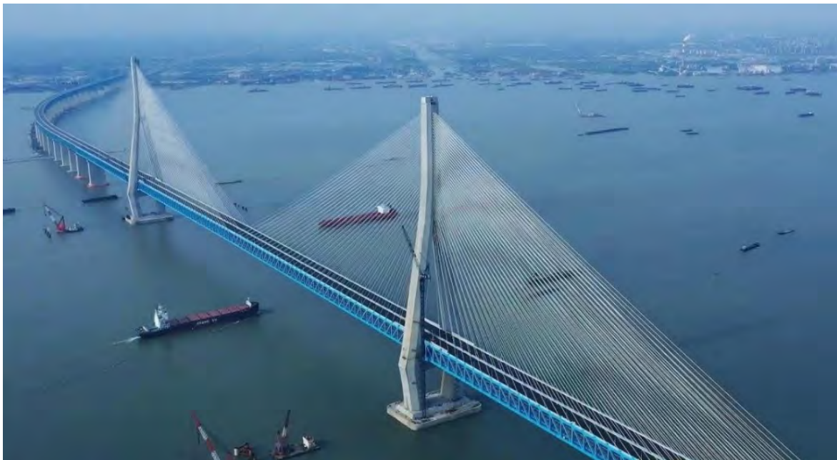
Figura 5-20 Hutong Yangtze River Bridge 137
