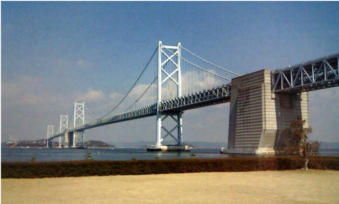
Figura 5-19 Minami Bisan-Seto Bridge 136
