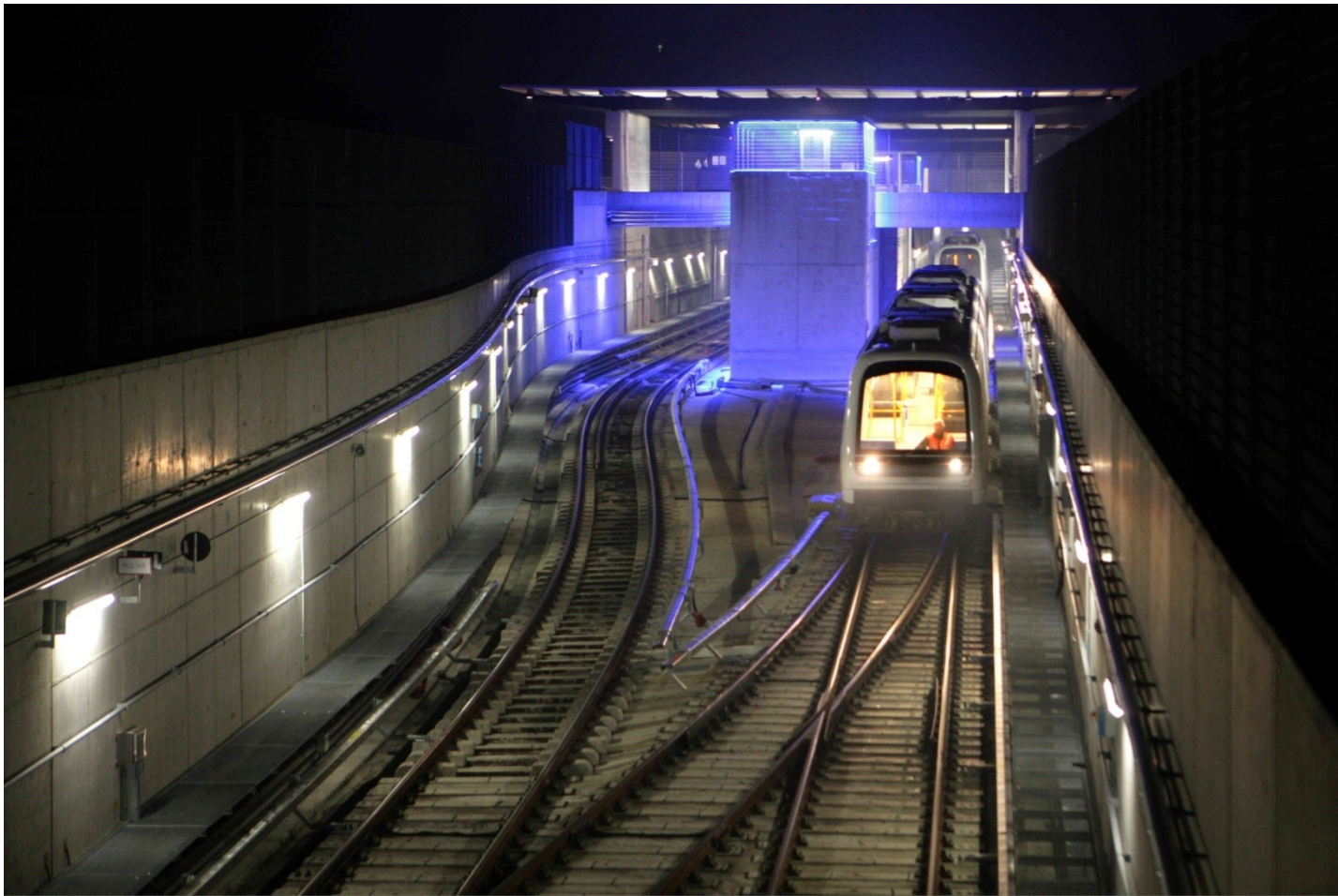
Metro Brescia – galleria c.a.
