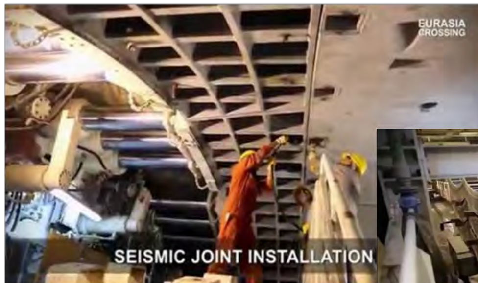
The Eurasia Undersea Tunnel Project
