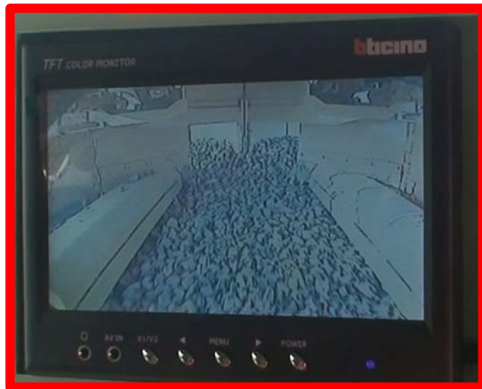
Monitor telecamera vomeri centrali
